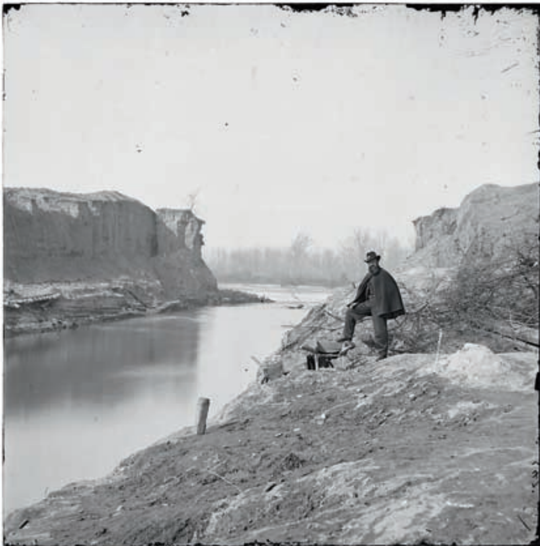
DUTCH GAP, VA. VIEW OF COMPLETED CANAL, 1865. STEREOGRAPH
